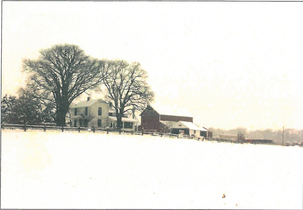
Blackberry Creek Farm, a Kane County Landmark
